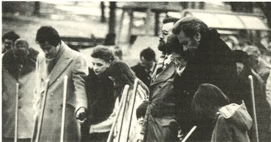
President Roberts, family, and supporters lift up the City of Faith project in prayer before breaking ground.
